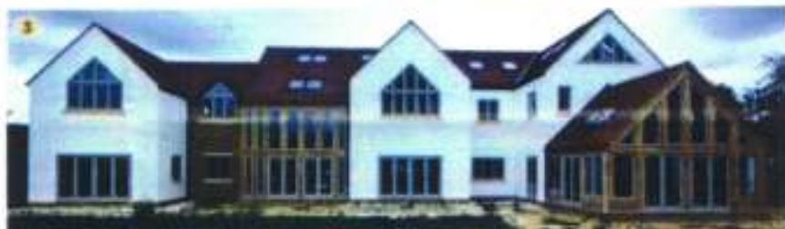
1 Croxfords was commissioned to create bespoke floor-to-ceiling timber framed glazing for this stunning rear extension. The bi-fold doors and tilt-and-turn windows are all idigbo hardwood framed with a factory-sprayed finish. 2 This brick and tile-hung house has been kitted out with windows and folding sliding doors from Timber Windows. 3 From French doors to triangular gable lights, this contemporary home shows the vast array of glazing options available from bespoke specialist, Meer End
